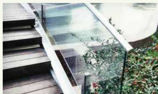
Bespoke steel bridge balustrade (above)
