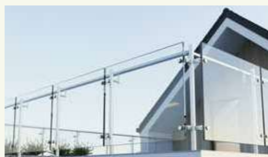
Supported external balcony extension (above)
